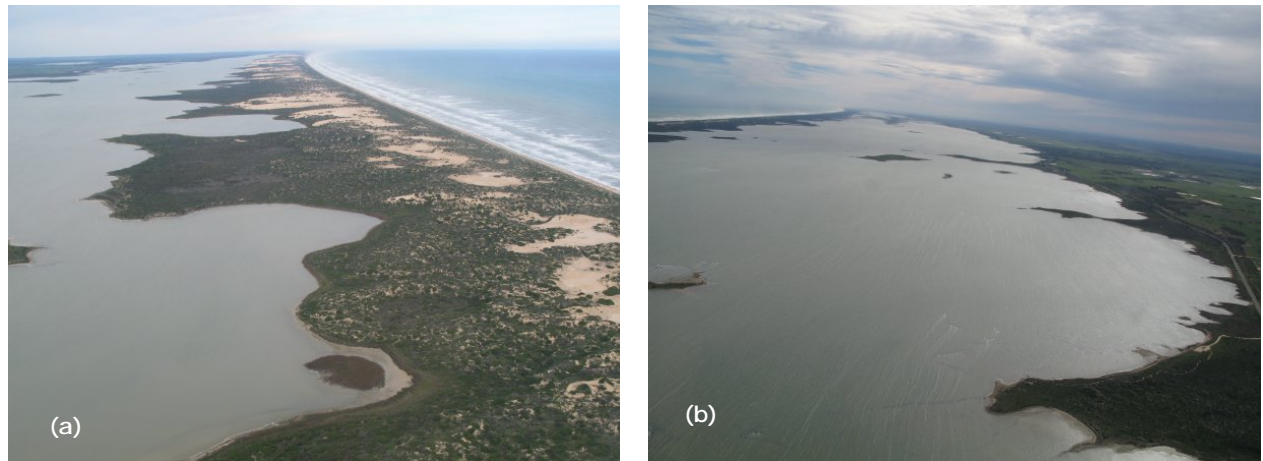
Figure 8. Aerial views of potential pumping infrastructure locations on (a) Younghusband Peninsula and (b) the eastern side of the South Lagoon.
